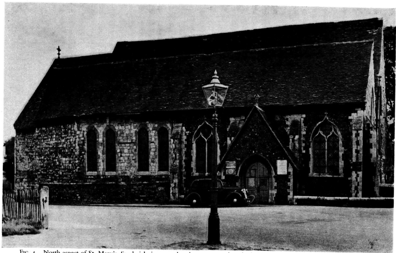
FIG. 4. North aspect of St. Mary's, Sandwich, in 1954, showing stone porch and rebuilt window to the left. (Compare FIG. 3.)
